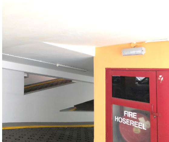
Emergency luminaire at each piece of fire fighting equipment and call point
