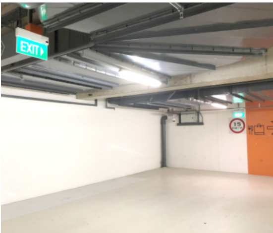
Directional exit signs at each change of direction and in areas where an exit is not readily available
